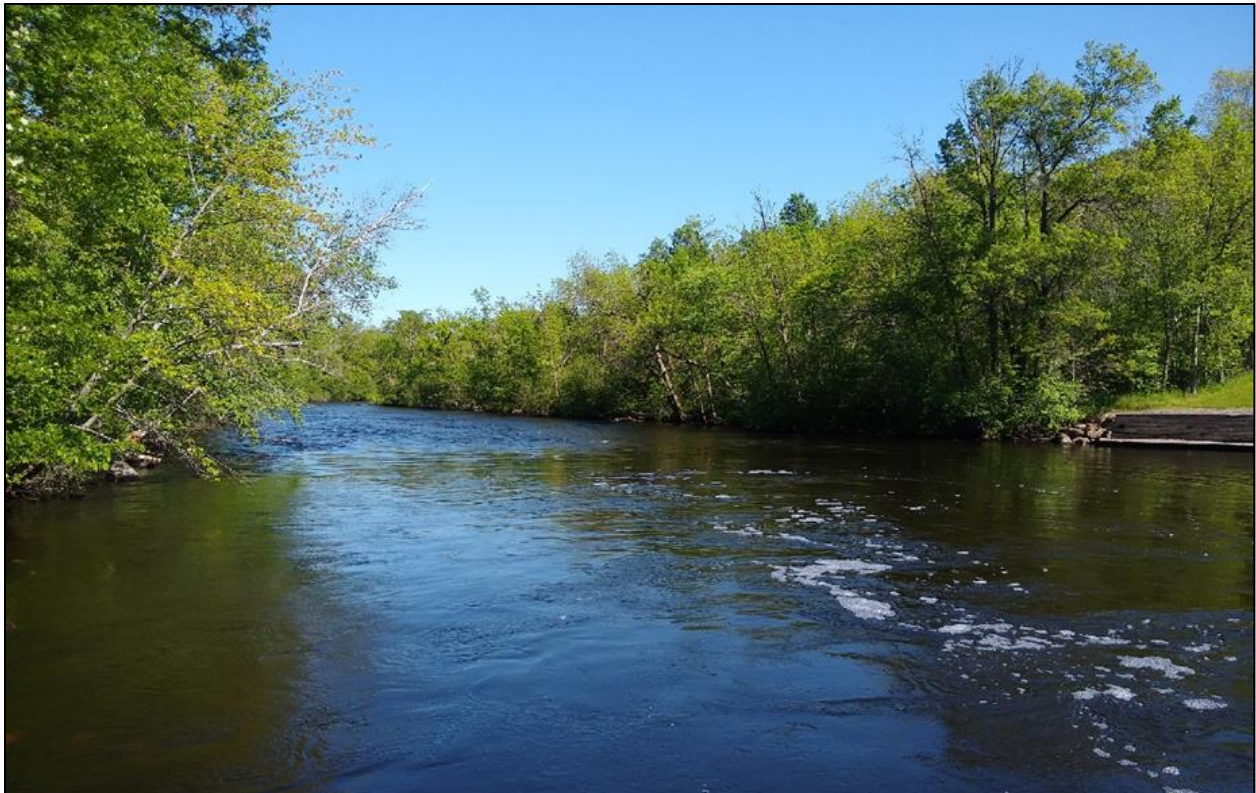
Figure 5.10.1-4 Downstream View of the Namekagon River from South Tailwater Fishing Area at the Trego Project
