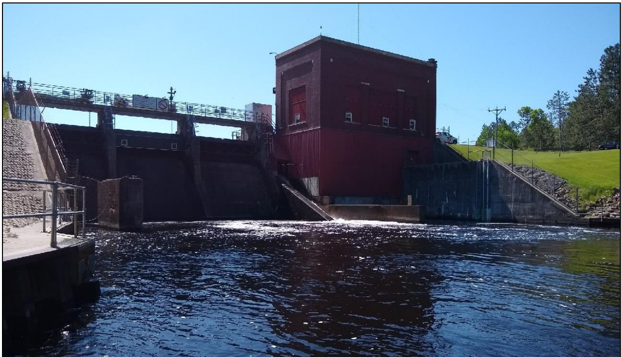
Figure 5.10.1-2 View of Trego Dam and Powerhouse from Canoe Portage Put-In (looking upstream)
