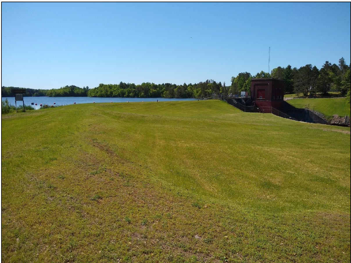
Figure 5.8.1.3.1-1 North Tailwater Access Canoe Portage Take-Out and Trail at the Trego Project
